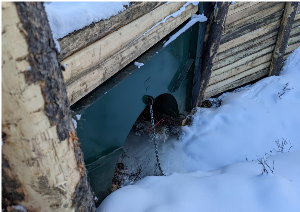
Figure 2. A reusable arch culvert installed on the Burnt Creek harvest.
