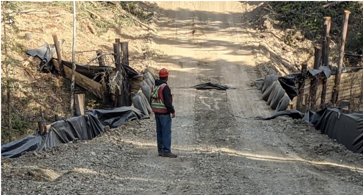
Figure 2. Temporary bridges with erosion controls are used across the forest
