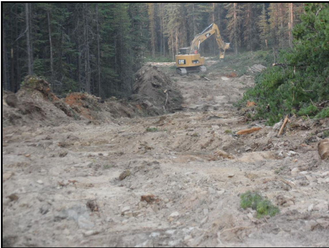
Figure 1. Road construction was inspected during the audit
